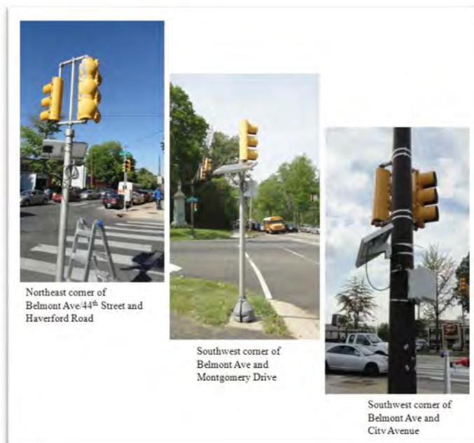
**Figure 1 – Typical Solar Powered BlueTOAD™ Device Installation**
